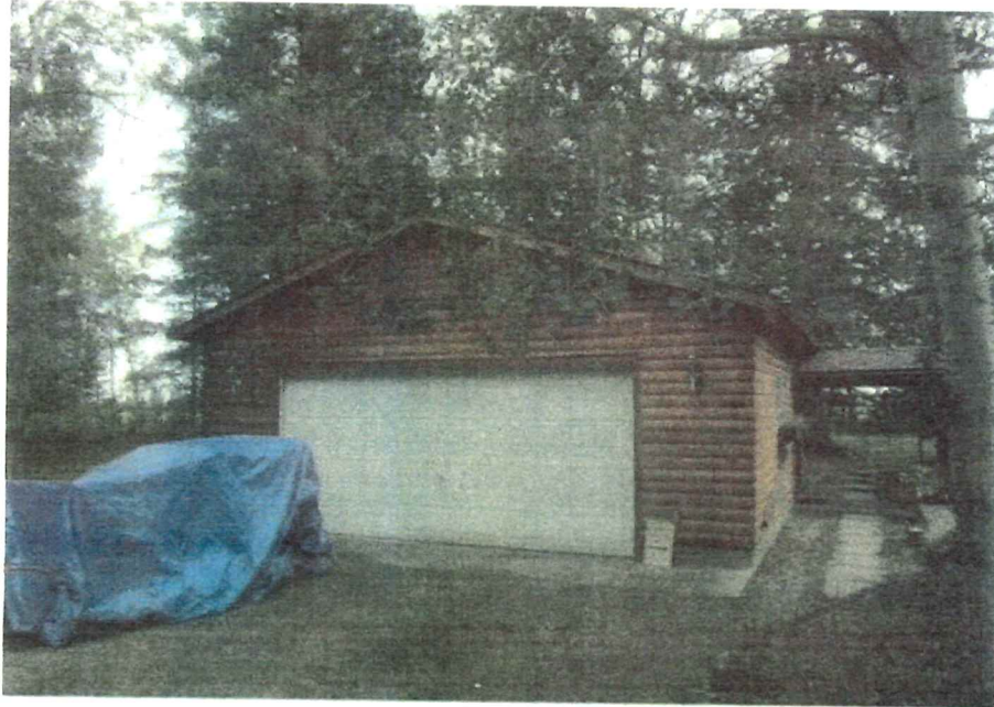
VIEW OF THE GARAGE NE-3
